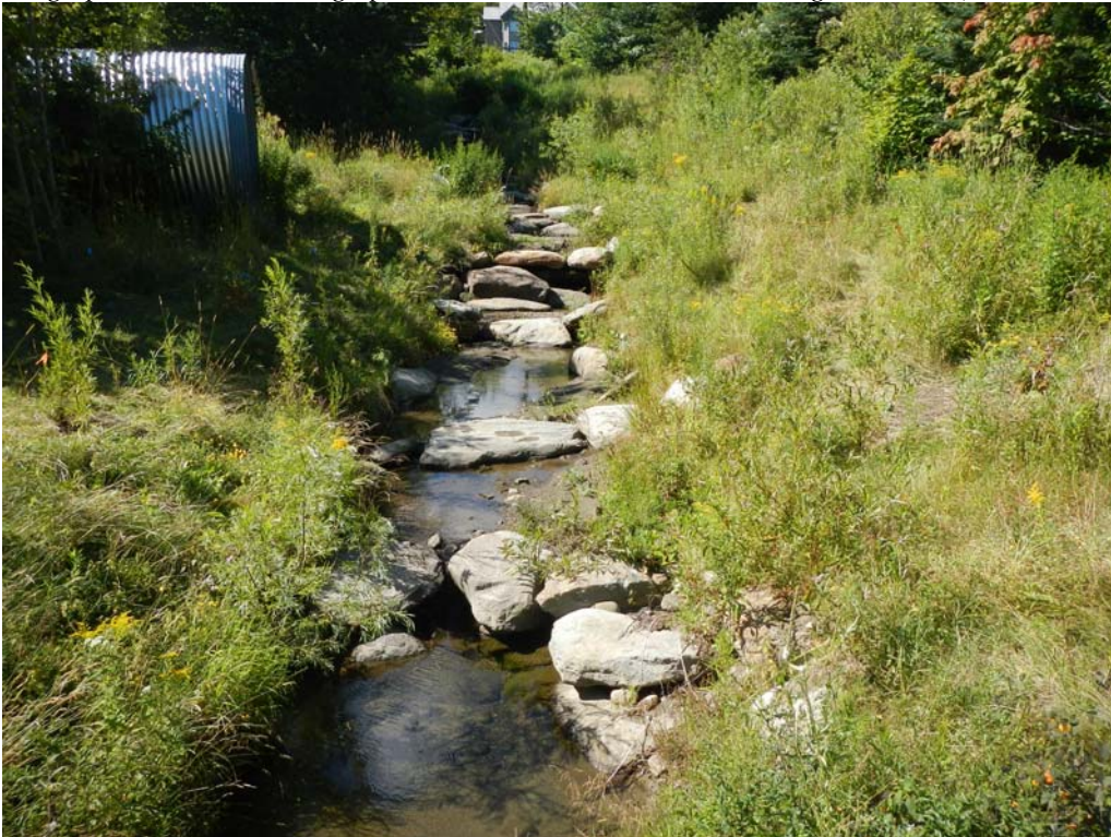
Photograph 20: P2-TB1 looking upstream from Station P2-TB1-P3, facing southwest (P. Werts, 8/15/13)
