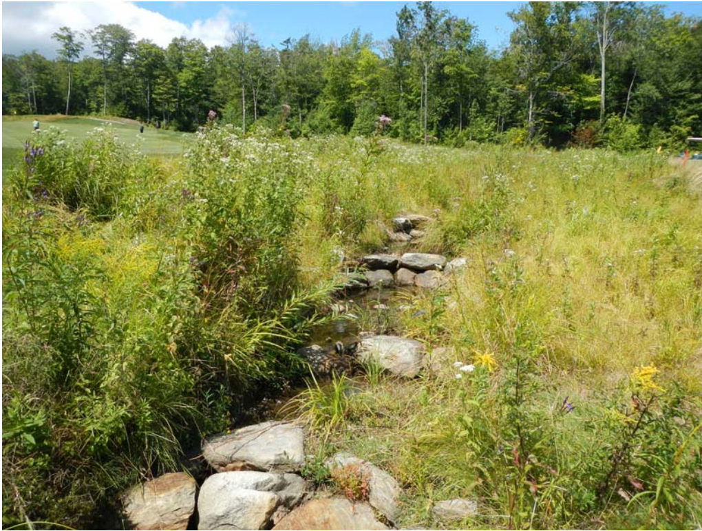
Photograph 7: H6-TB1 from Station H6-TB1-P2, facing northwest (P. Werts, 8/15/13)
