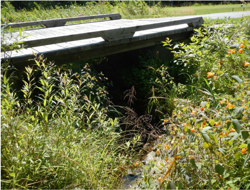
Photograph 1: H5-TB3 from Station H5-TB3-P1, facing east (P. Werts, 8/15/13)
