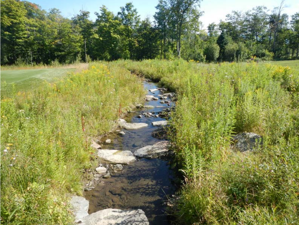
Photograph 18: P2-TB1 looking downstream from Station P2-TB1-P1, facing northeast (P. Werts, 8/15/13)
