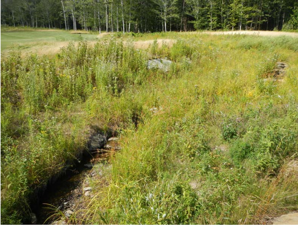
Photograph 25: H11-TB2 from Station H11-TB2-P1 facing north (P. Werts, 8/15/13)
