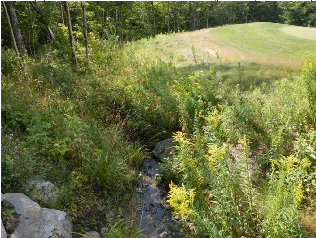
Photograph 38: H15-TB1 from Station H15-TB1-P1, facing south (P. Werts, 8/16/13)
